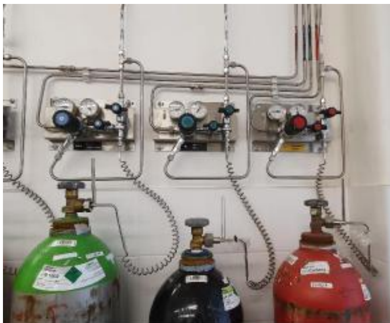
Figure No. 15: Pressure regulator on a wall-mounting plate
